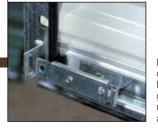
Dual 12-gauge, zinccoated interior steel latches slide into door guide brackets. Latches may also be padlocked for added security.
